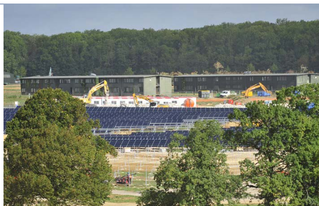
Toul project (France)
