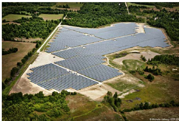
Saint-Isidore B (11.8 MWp in Canada)
