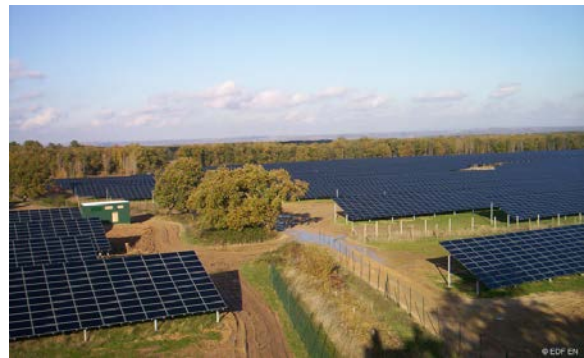
Bouloc (10.2 MWp in France)
