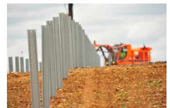
pose des structures
